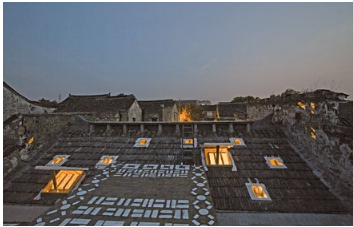
Forty traditional-style skylights lead to a 'hall' under the sloping roof and the sky. Walking out from a window and standing on the little platform, one is totally embraced by hills of grey tiles.
